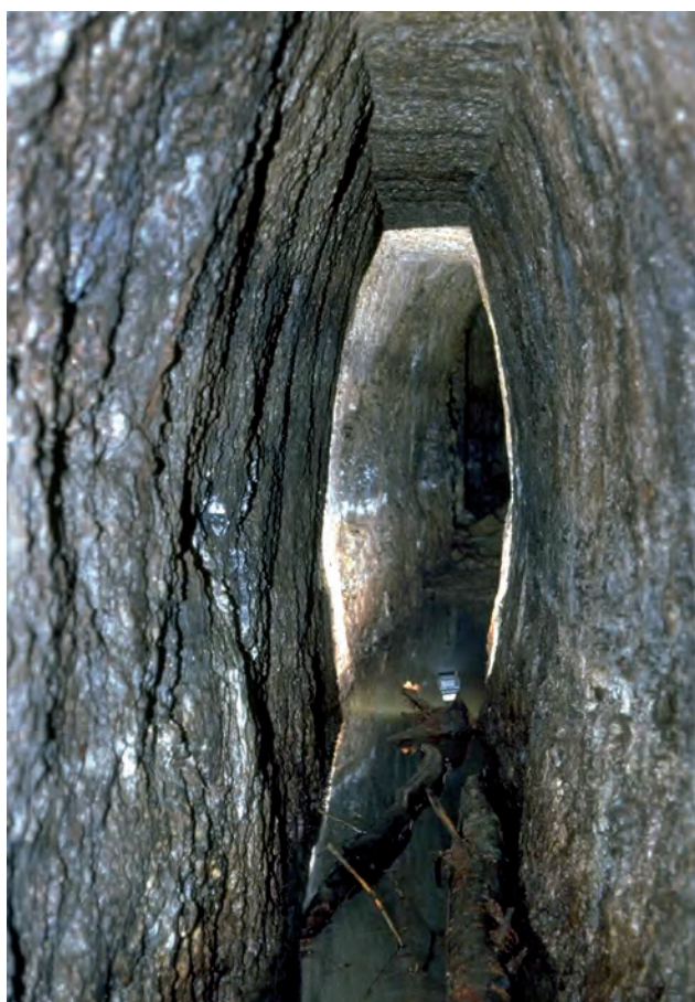
Fig. 17 - Bartholomäberg, Montafon. View of an adit (Schrämmstollen) hewn into the bedrock in the area of medieval mining activities, Knappagruaba parish (cf. map Fig. 3).
